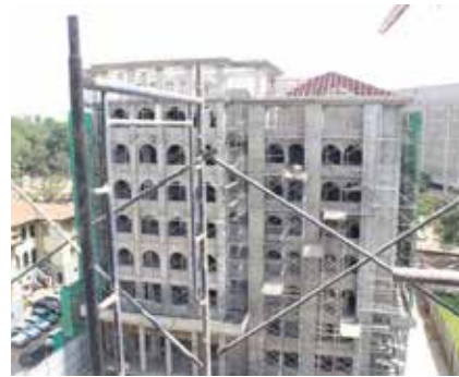
ON COURSE: Progress on the construction of Appellate Courts
